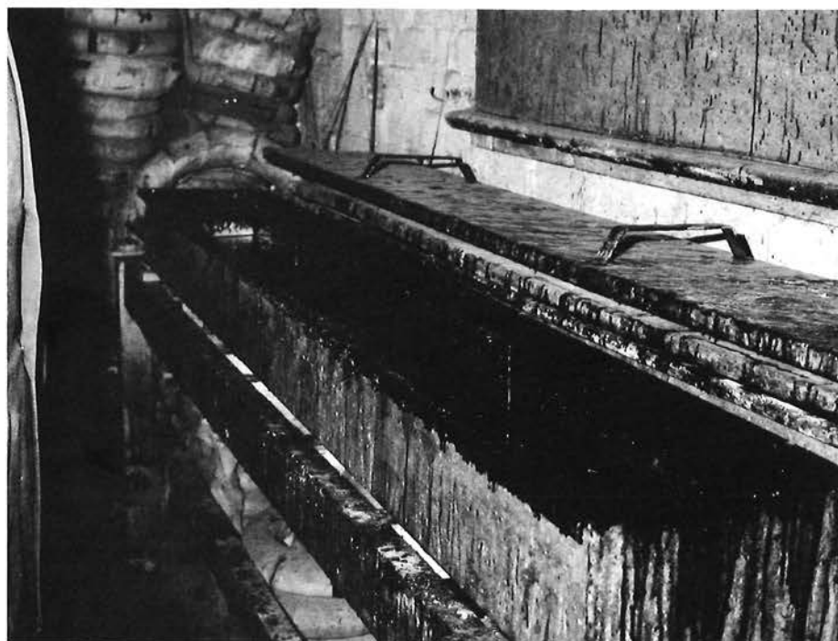
Above: The resin tank.
